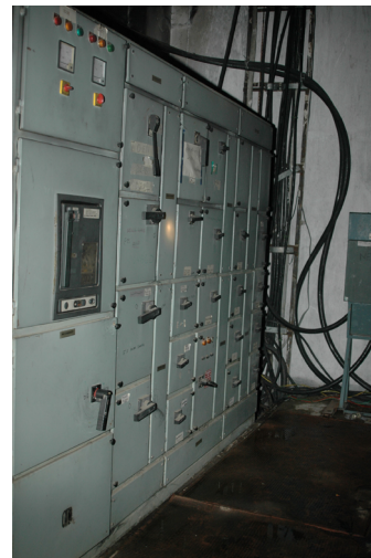
Figure 3: showing distribution circuit were intact.
